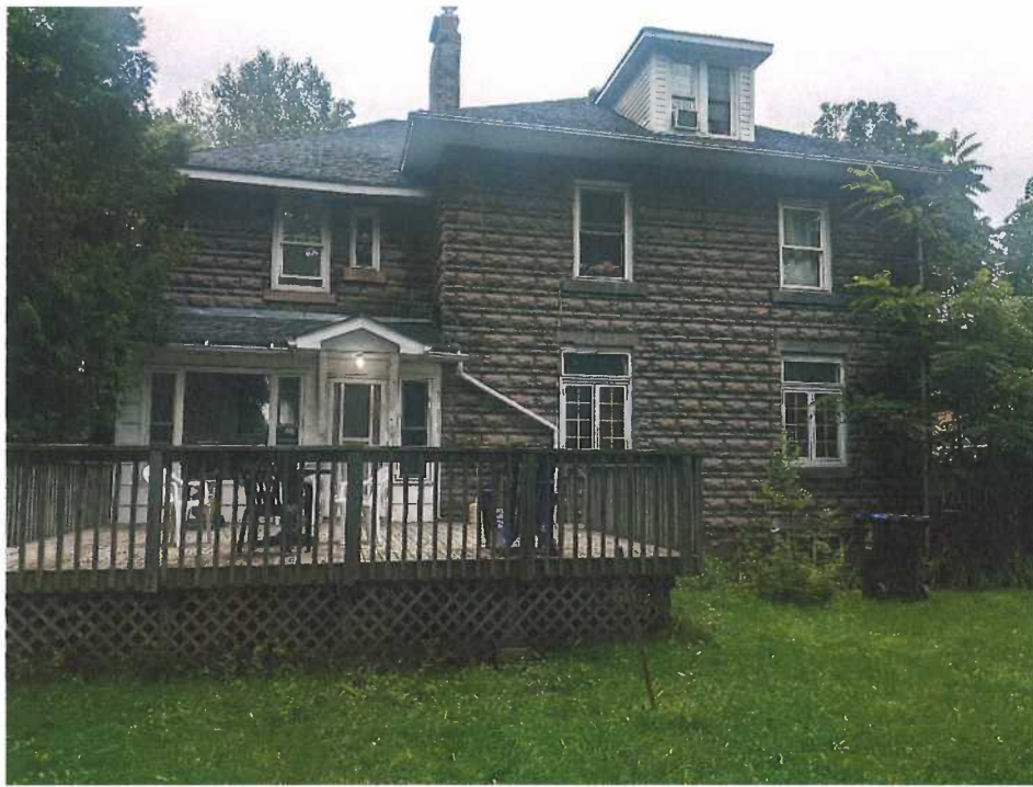
Photo: North-West Elevation (Rear of House)
