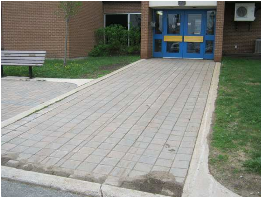
G203003e - Interlocking Brick at Front Entrance
