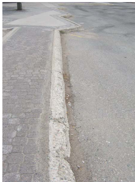
G202002 Scraped and scaled curbs
