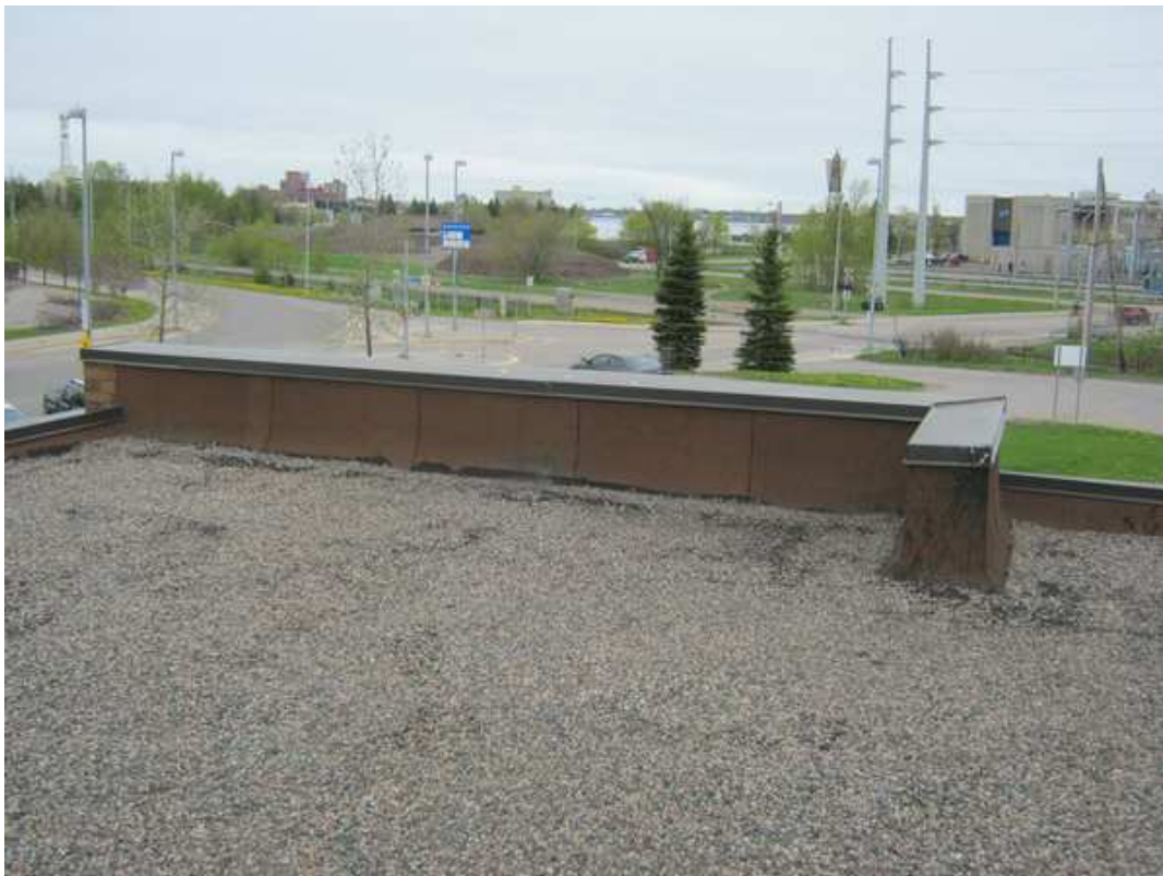
B3010a Newer Built Up Roof over office with Modified Bitumen Flashings
