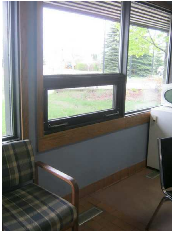
B2020 Typical Window, showing newer operable unit
