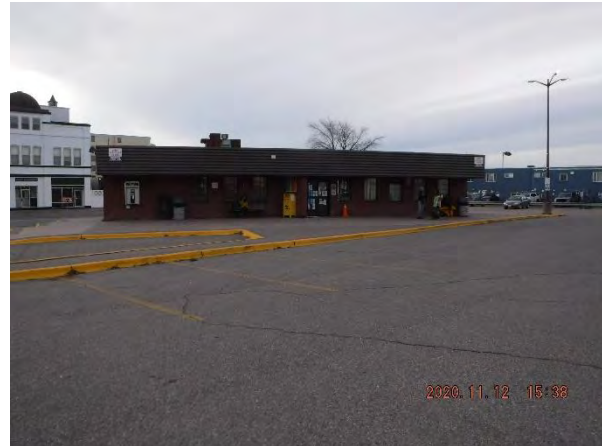
Photo 2 - Existing transit terminal and parking area.
