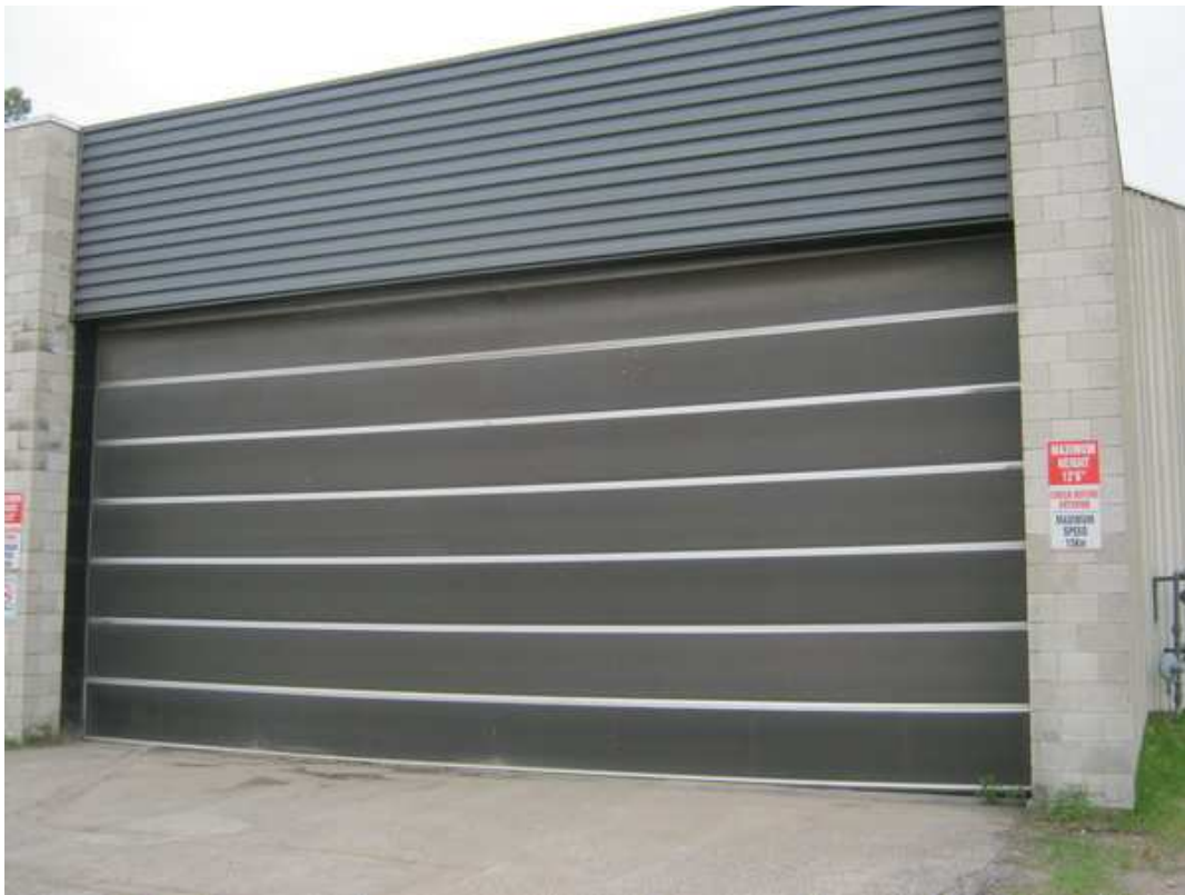
B203004b Main Garage Entrance Door from Huron Street
