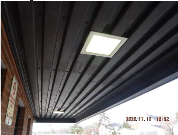
Photo 3 – Structural overhangs of the existing transit terminal.
