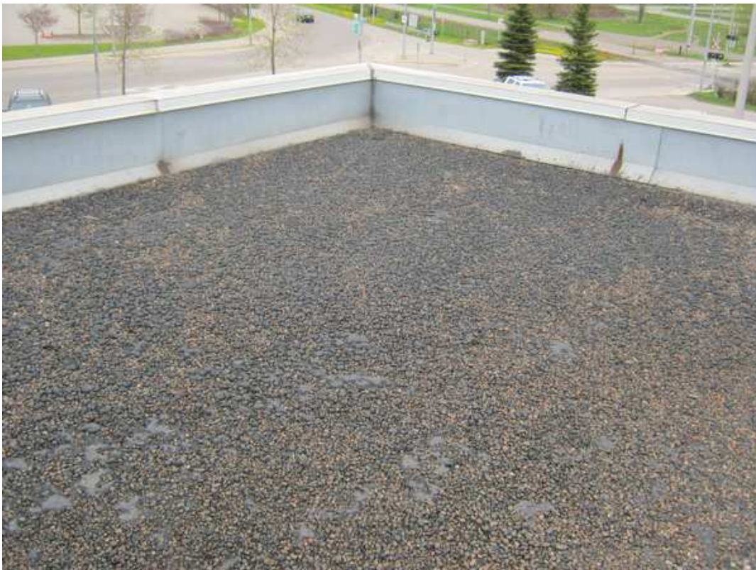
B3010c Blueberries, or pockets of roofing pitch suggesting an aged roof
