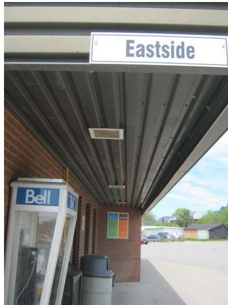
D502002 Soffit mounted exterior lighting
