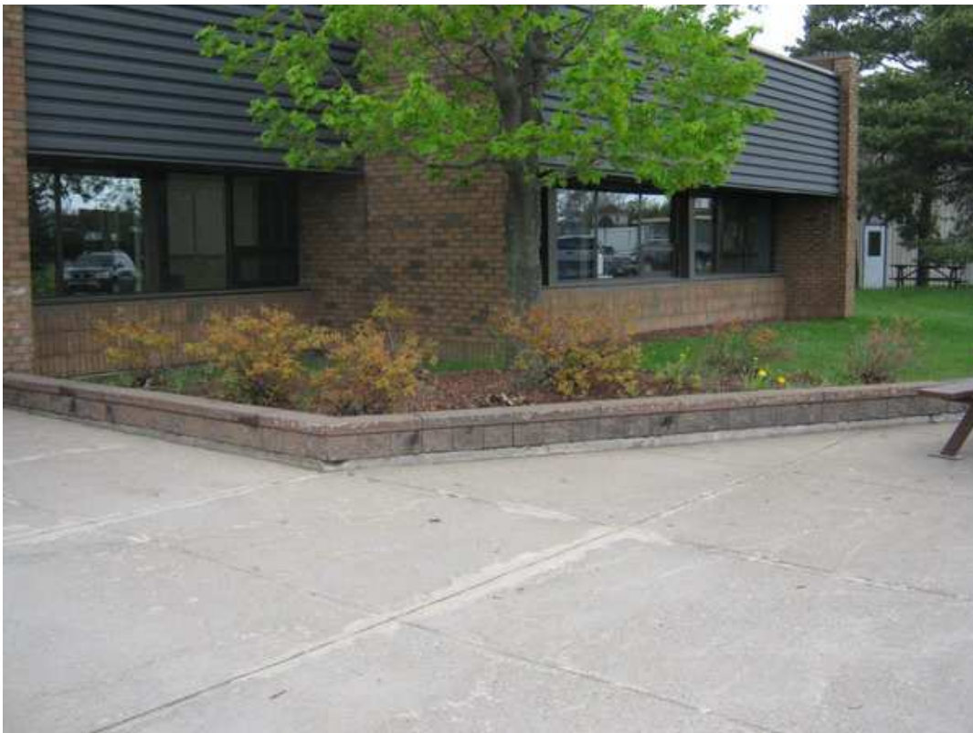
G202002 Overview of Concrete Sidewalk
