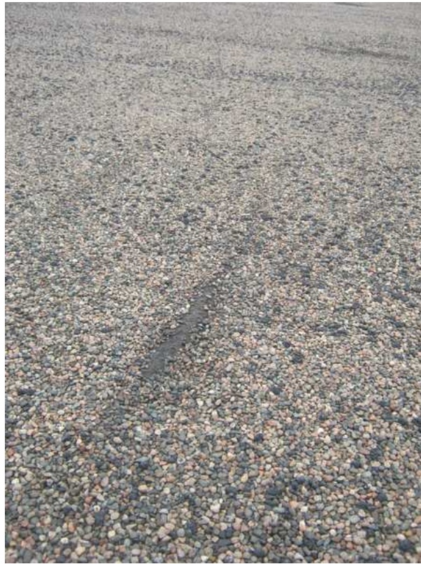
B3010b Typical Ridging and Exposed Felts at Garage Roof
