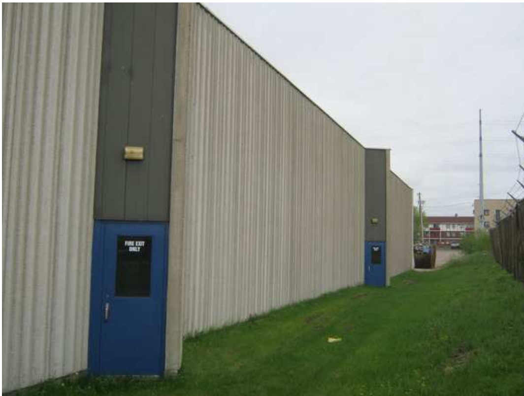
D2010a Overview of Precast Concrete Cladding
