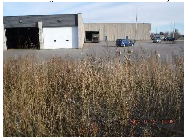
Photo 6 – Parking areas and errant grasses at the northwest side of the Transit Services Facility.
