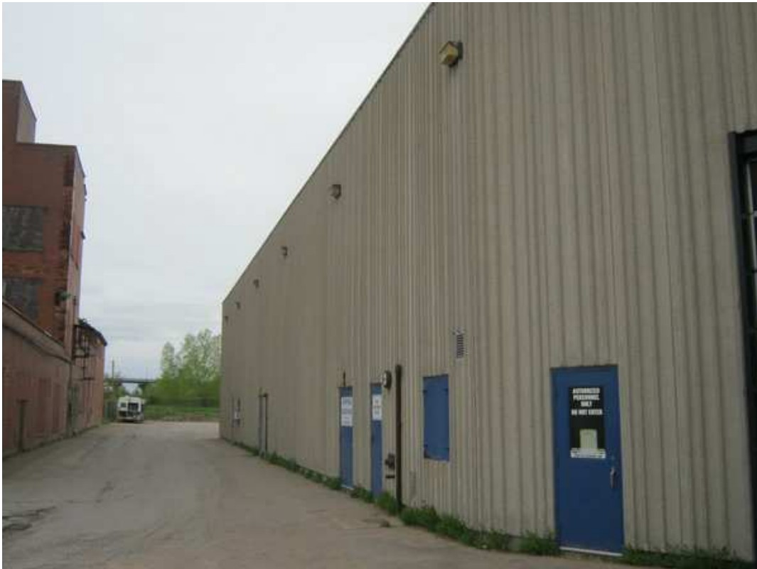
G203003d Pavements adjacent to neighbouring building assumed to be part of this property
