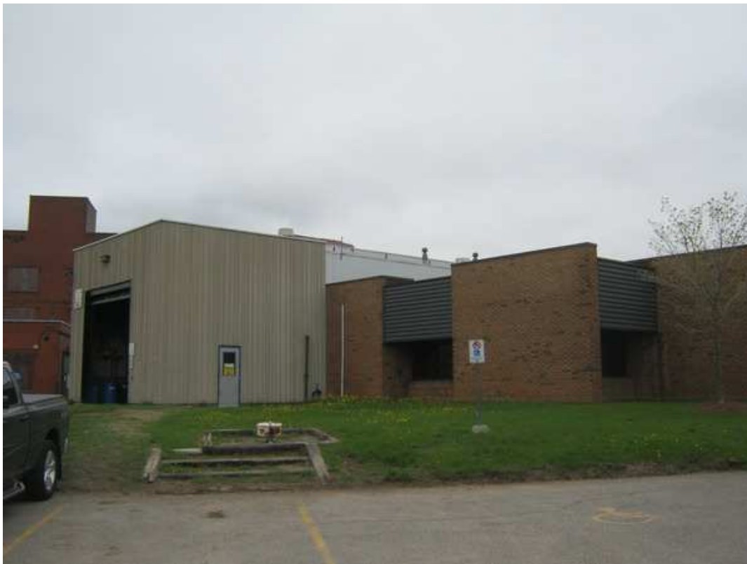
A0 Building Overview
