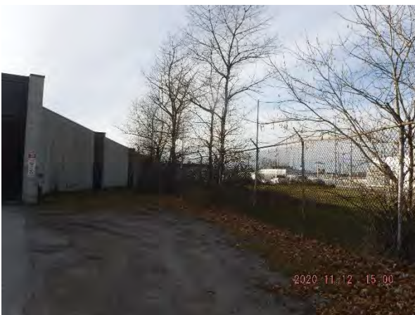
Photo 5 – Northern edge of the Transit Services Facility (most likely area at this Site that is being considered for new terminal).
