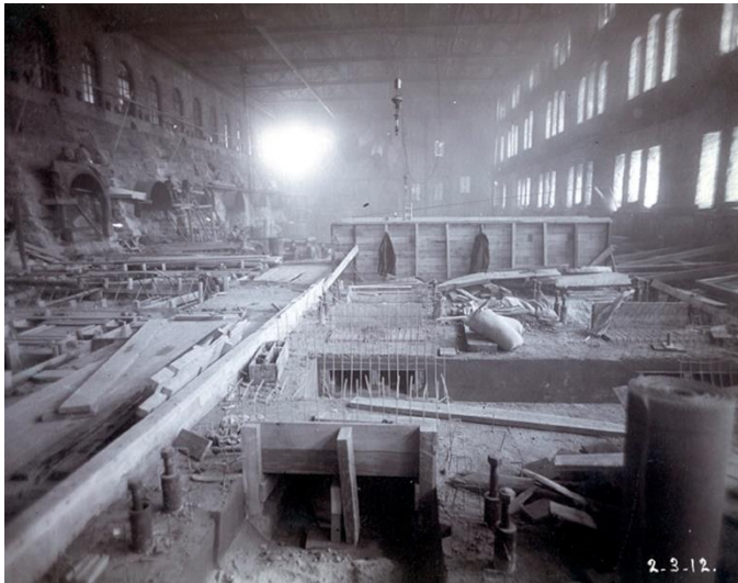
Interior view of the Machine Shop while under construction. Year: 1895-1901. Source: Sault Ste. Marie Museum / Community Stories at Virtual Museum of Canada.
