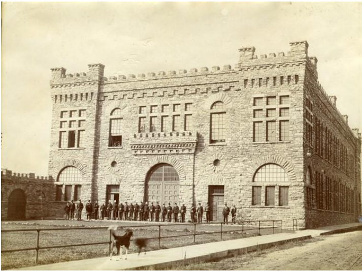
The Machine Shop building completed. Year: unknown. Source: Sault Ste. Marie Public Library.
