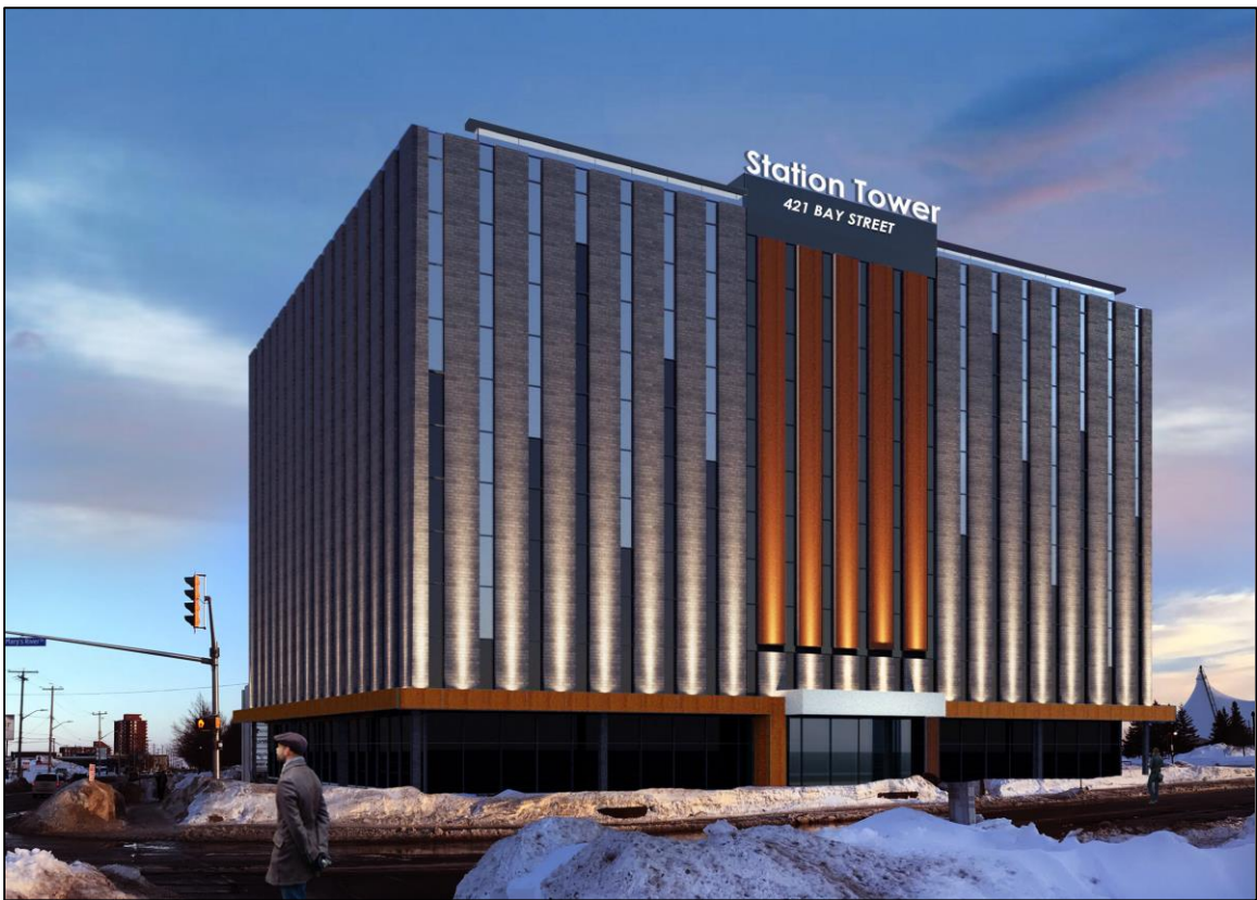
Façade Improvement: 421 Bay Street
