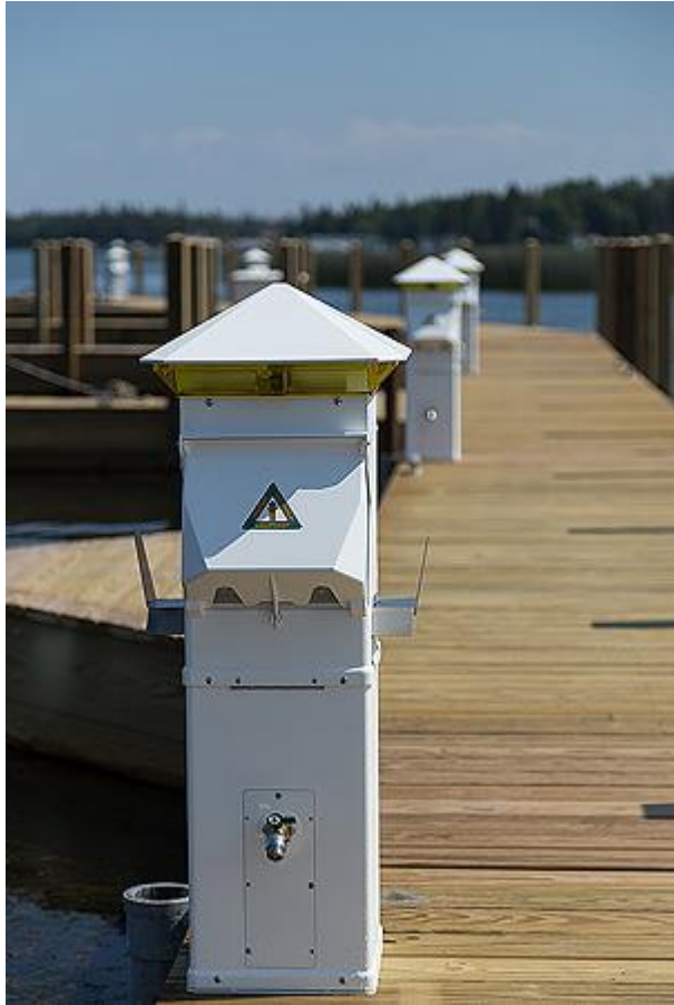
Fig 5.- Pedestals (23) – 30 amp double sided (2 reused) – electrical supply in existing panels assumed to be sufficient for current layout
