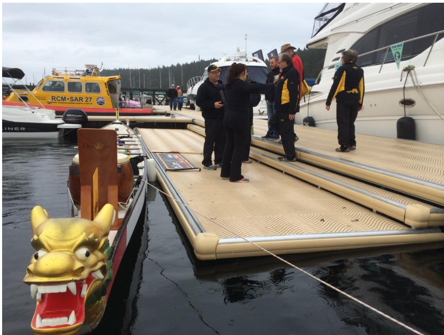
Figure 3 - Example of a low-profile dock – one section of dock is planned to be low profile in the marina to enable easier access for canoe/kayaks, etc.
