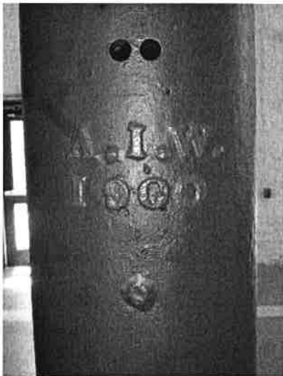
Cast Iron Interior Column
