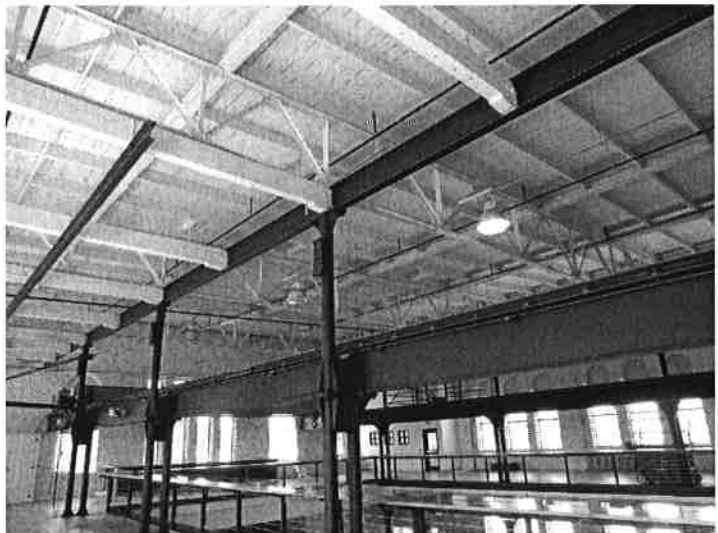
Mezzanine Level Floor
