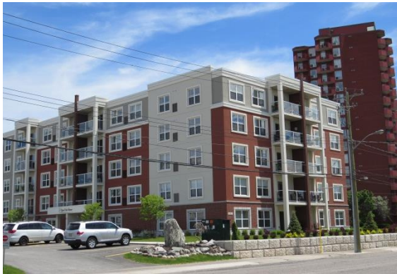
River Park Manor Apartments, 676 Bay Street
