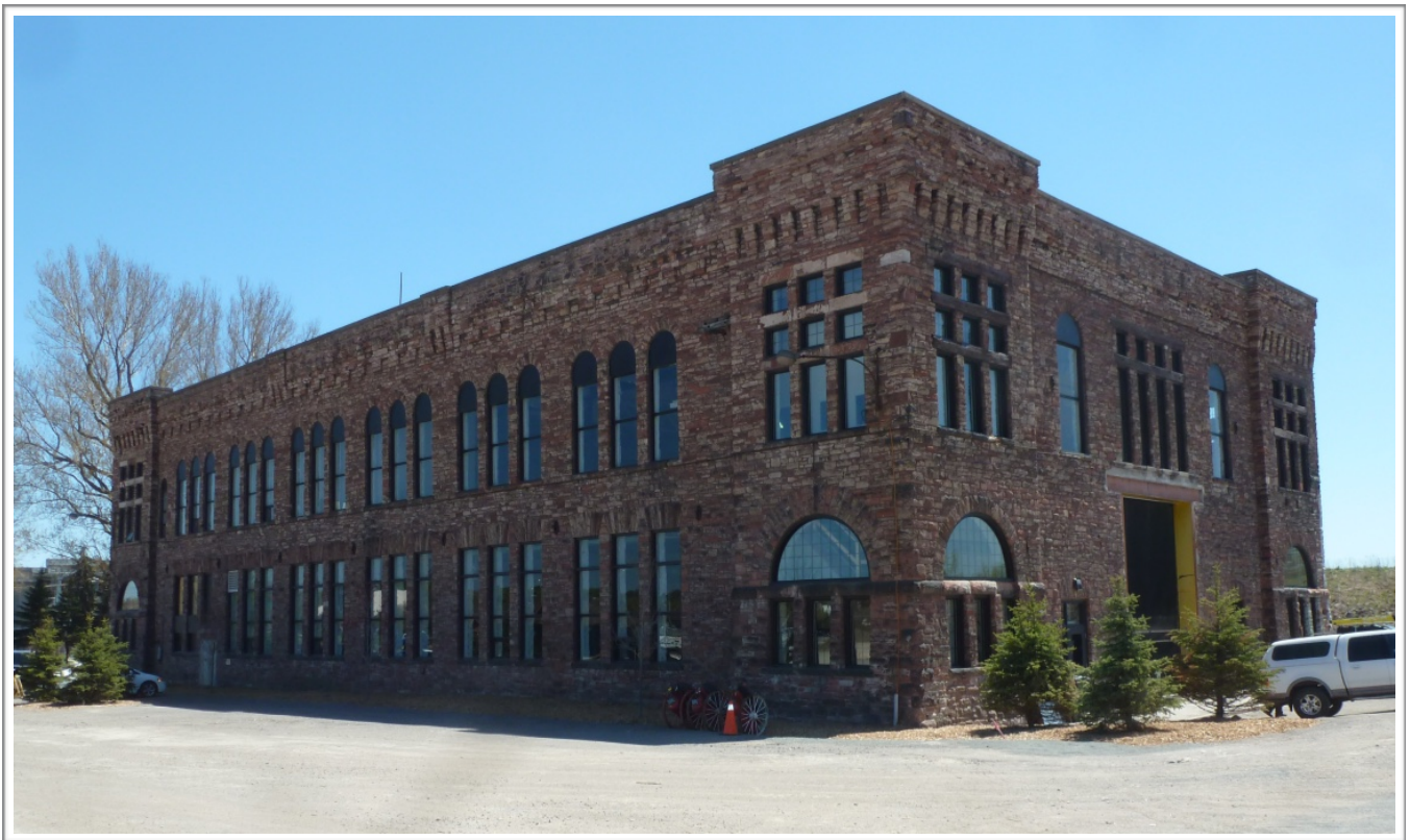
Machine Shop - North-West Elevation
