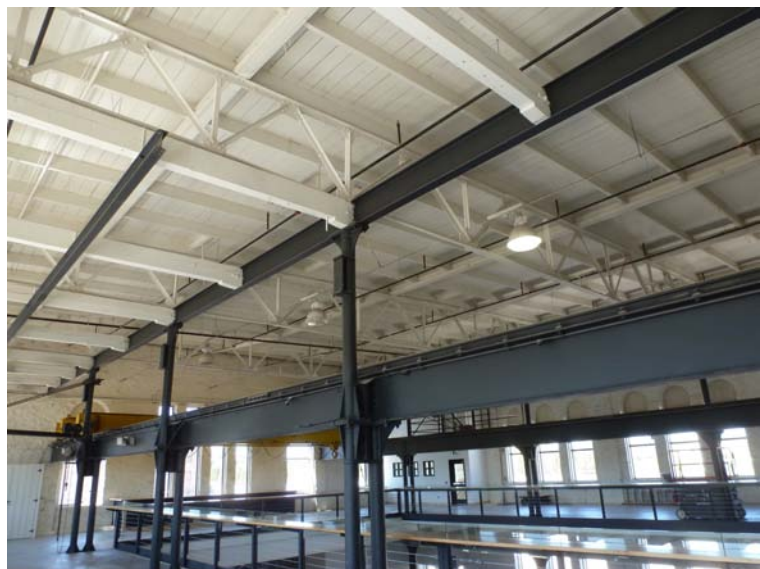
Mezzanine Level Floor
