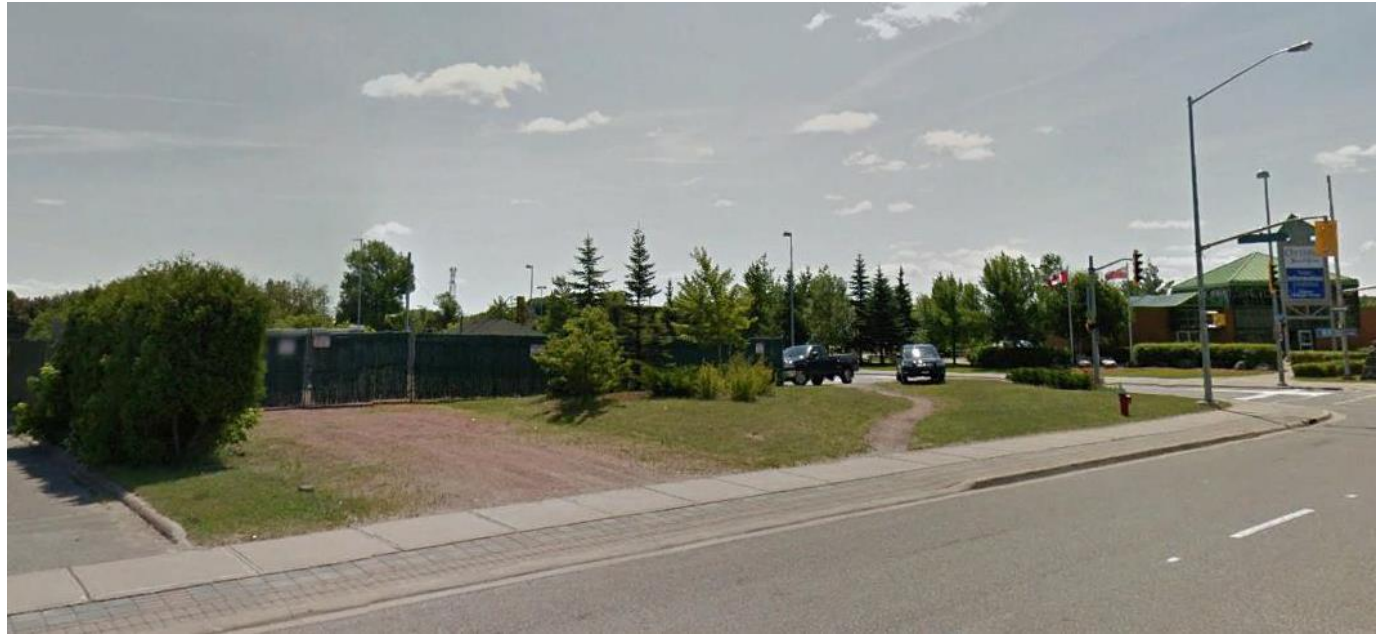
Welcome Feature Site: Northeast Corner of Huron Street and Queen Street West, currently a PUC Substation
