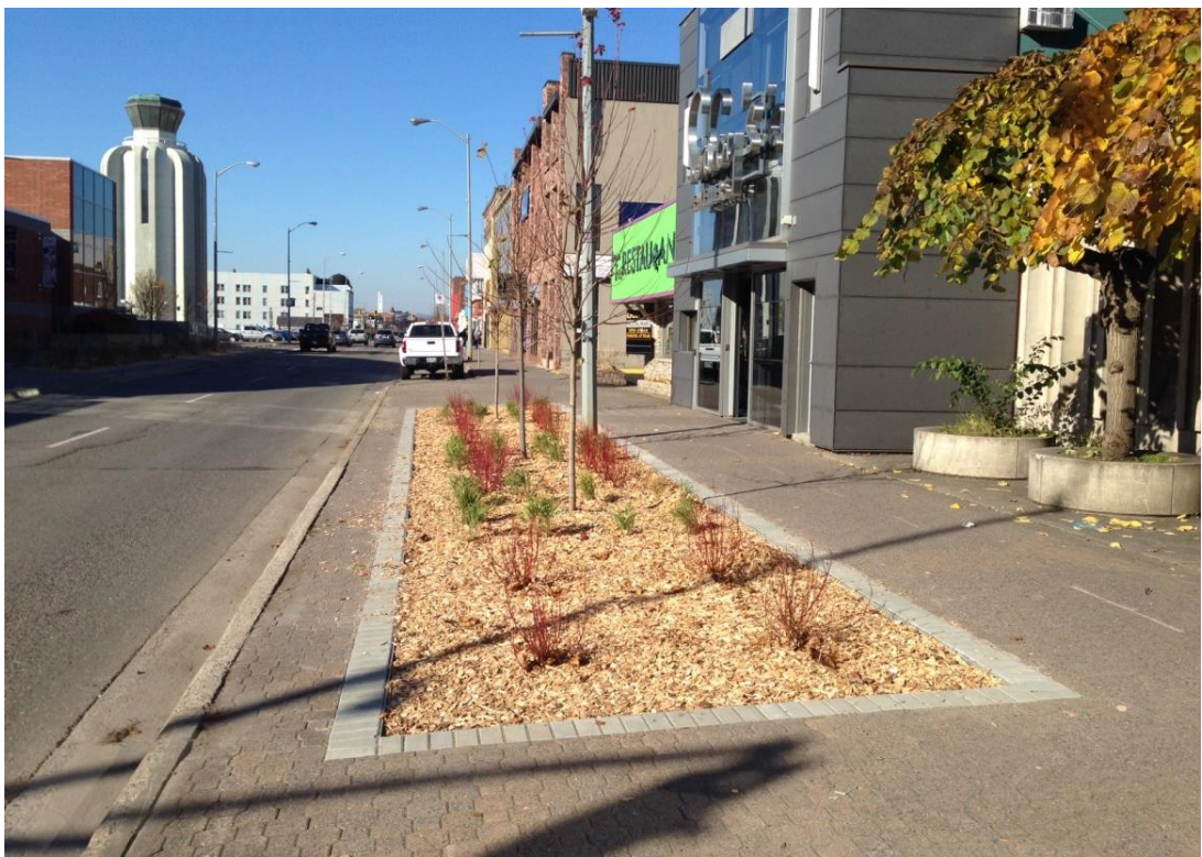
Root Trench System Implemented between Dennis Street and Bruce Street
