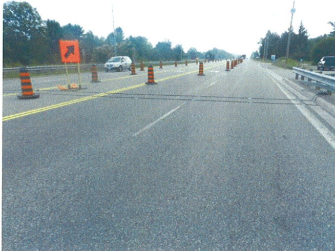
Eastbound Approach (View East)
