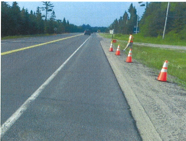
Southbound Approach (View South)
