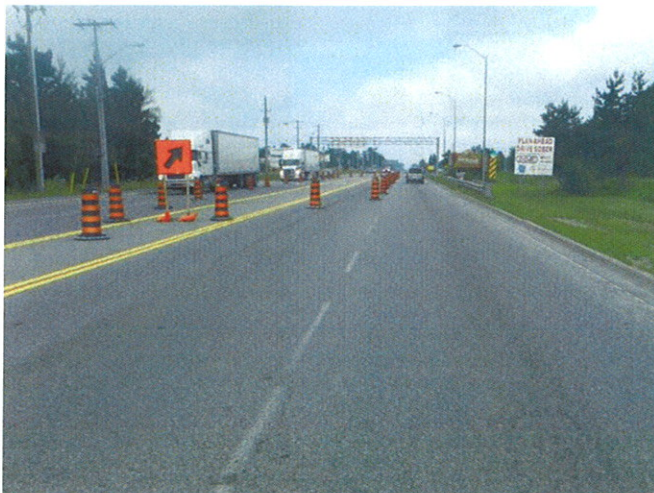
Westbound Approach (View West)
