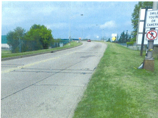
Westbound Approach (View West)
