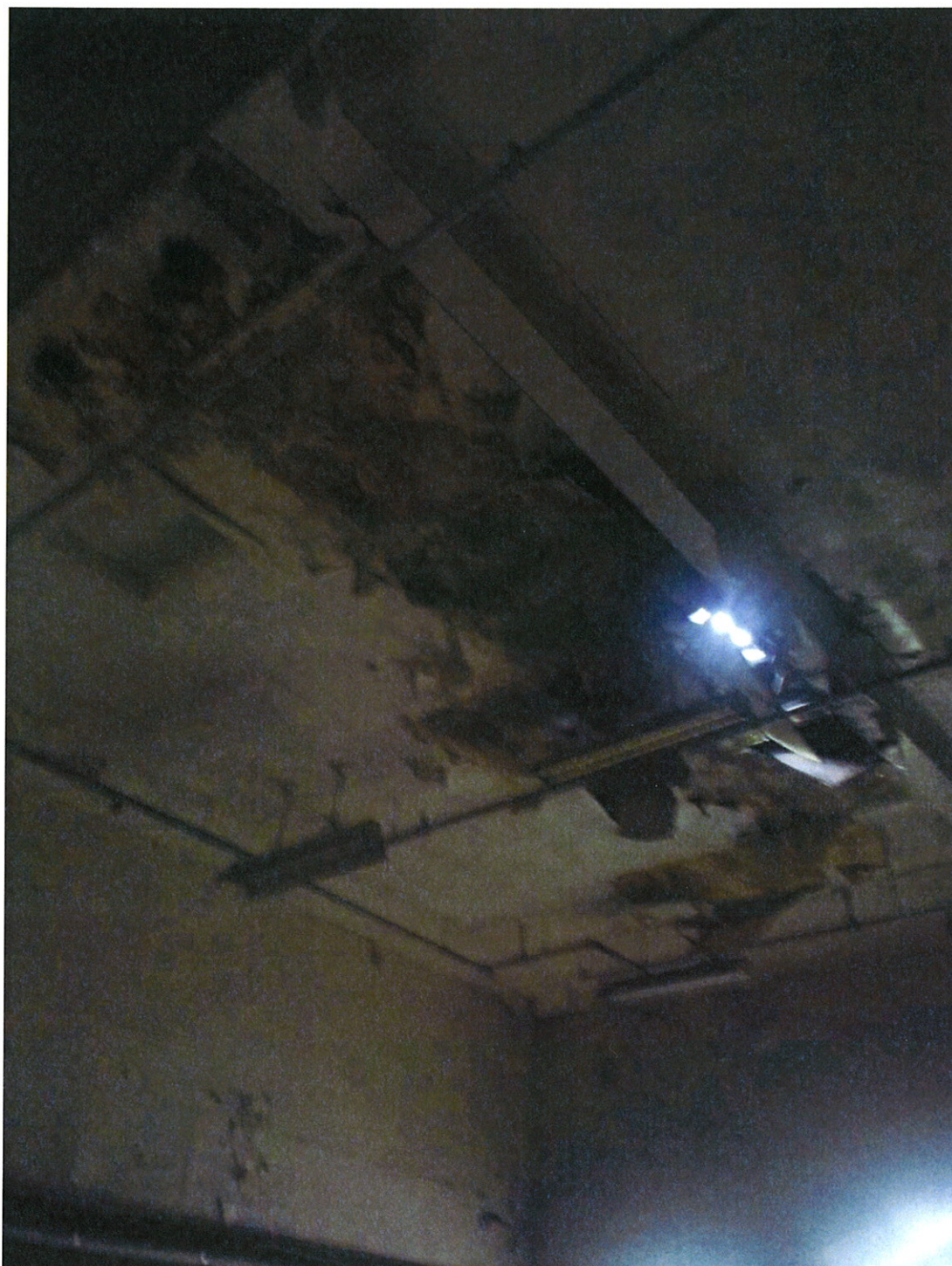
Photo No. 2 Roof Penetration No. 2
