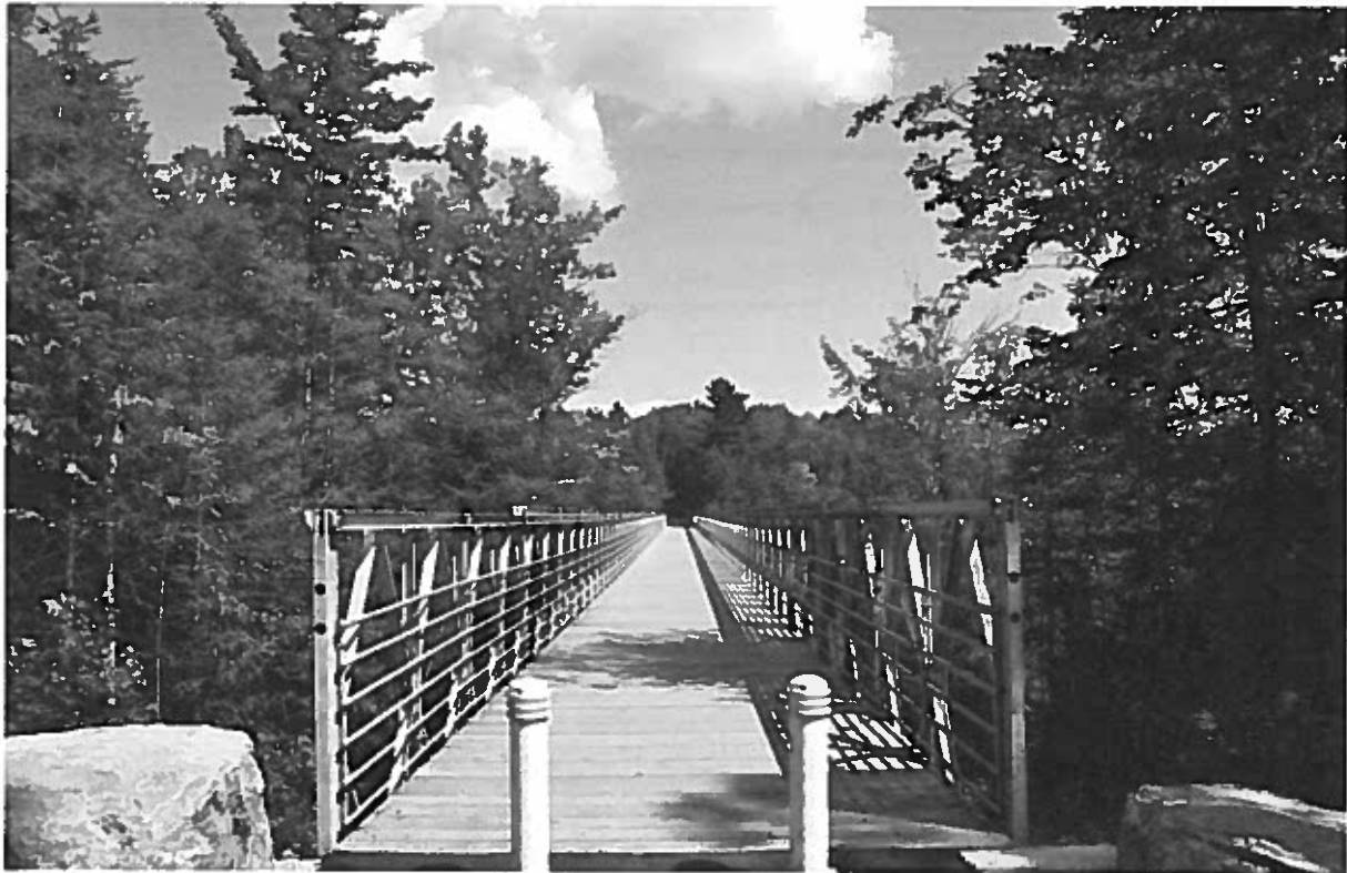
John Rowsell Hub Trail @ Fort Creek
