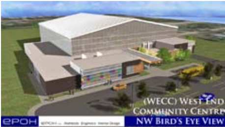
The soon-to-be built West End Community Centre.
