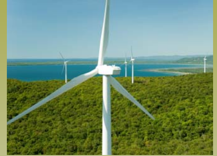
The Prince Wind Farm
