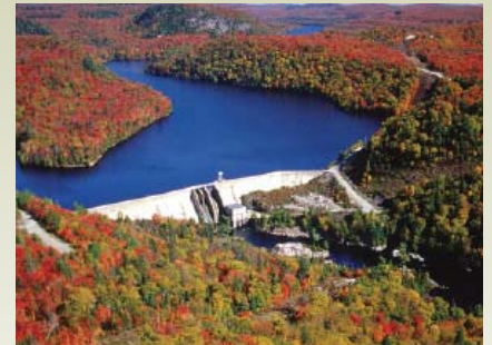
Montreal River Hydroelectric Station
