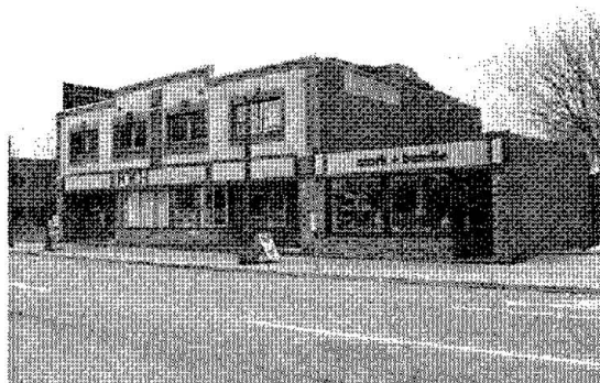
Foch's Cleaners (721 Queen Street East) – After Construction
