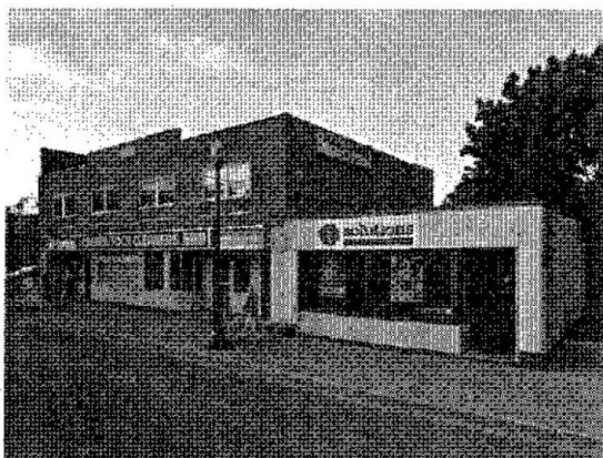
Foch's Cleaners (721 Queen Street East) – Before Construction
