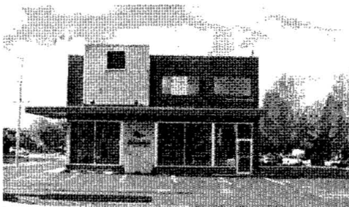
Chamber of Commerce (489 Bay Street) – After Construction
