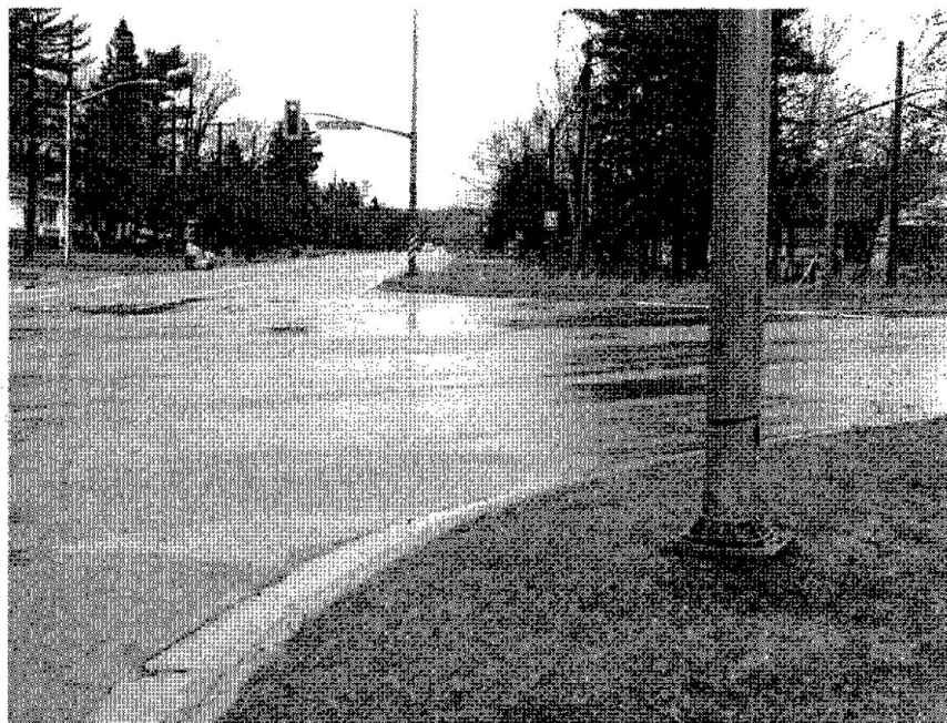
East side of Old Garden River Road/Second Line West Intersection – No crossing signals exist for pedestrians or trail users to continue north
