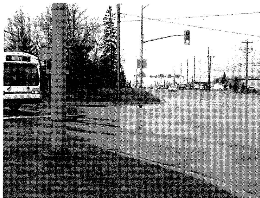
South side of Old Garden River Road/Second Line West Intersection – No crossing signals exist to allow south bound pedestrians or trail users to cross in order to access EMS Centre trail to the south
