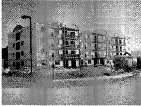
723 Bay Street – During Construction
