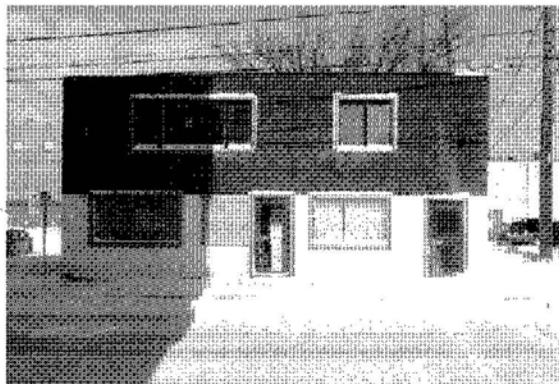
67 Elgin Street – Before Construction
